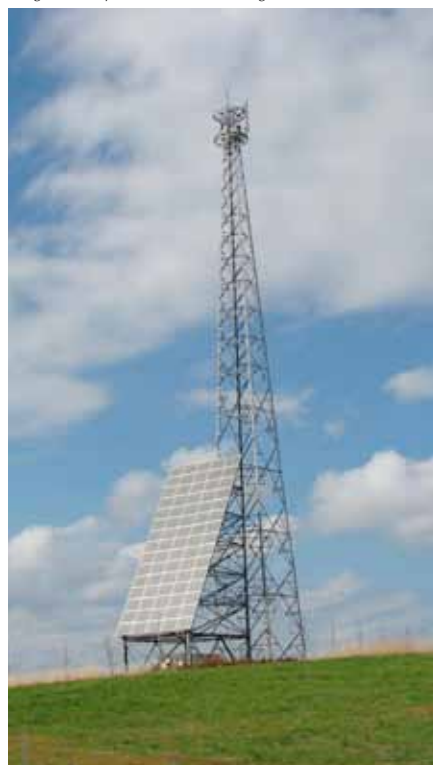
Mobile-phone base station powered by photovoltaics
