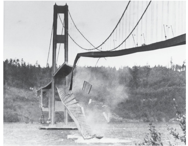
Fig. 9.2.7 The Tacoma Narrows Bridge collapsed in November 1940, as the result of resonant energy transfer between the wind and the bridge surface. Shortly after its construction, the automobile bridge began to exhibit an unusual natural resonance in which its surface twisted slowly back and forth so that one lane rose as the other fell. During a storm, the wind slowly added energy to this resonance until the bridge ripped itself apart.
